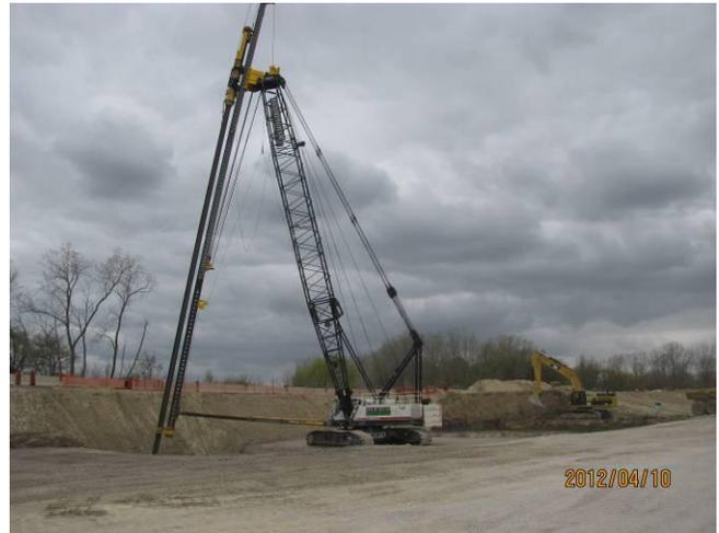
A diesel hammer pile driver at Bridge 10
