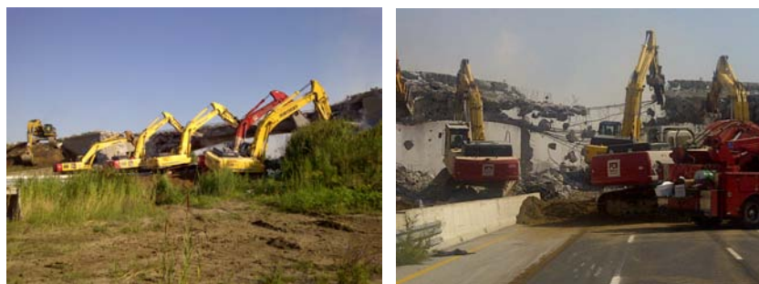
Left: Parkway crews work to remove the North Talbot Road Bridge over Highway 401.
