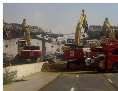
Left: Parkway crews work to remove the North Talbot Road Bridge over Highway 401.
